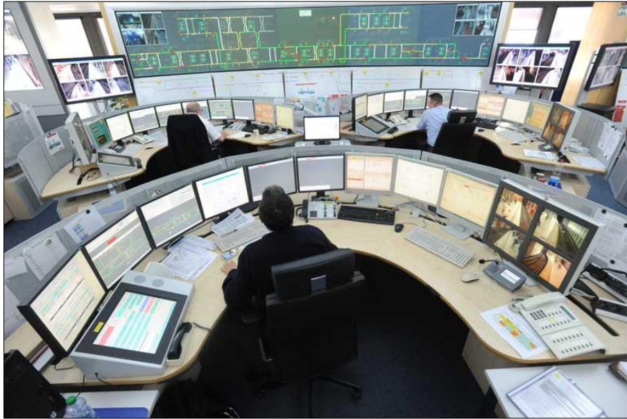
Figure 4: Monitoring the autonomous underground in Nuremberg from the control centre (© VAG – Claus Felix).
