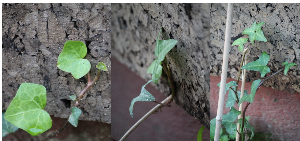
Figure 4. Ivy plants adhering to cork boards of the indirect green façade at Ajuda Botanical Garden, Lisbon, Portugal (February 2022).
