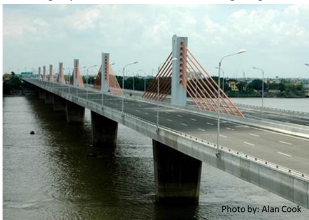
Figure 1: Second Vivekananda Bridge, India.
