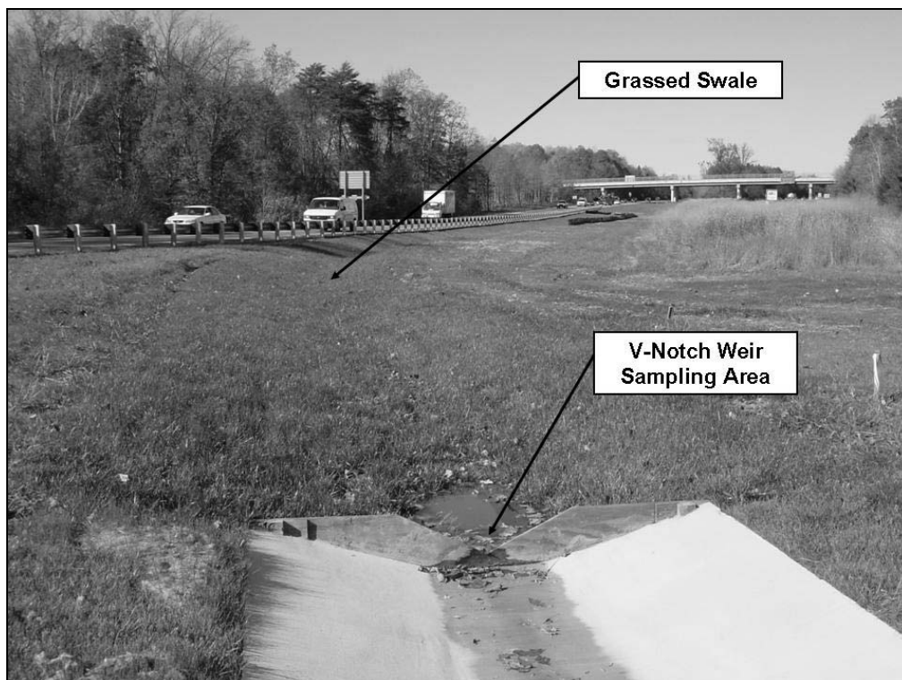
Figure 3-5. SHA swale at Rt 32.
