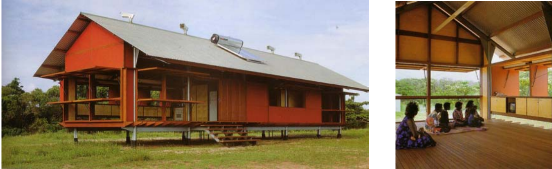
Figure 32: Exterior and interior photograph; Fromont
