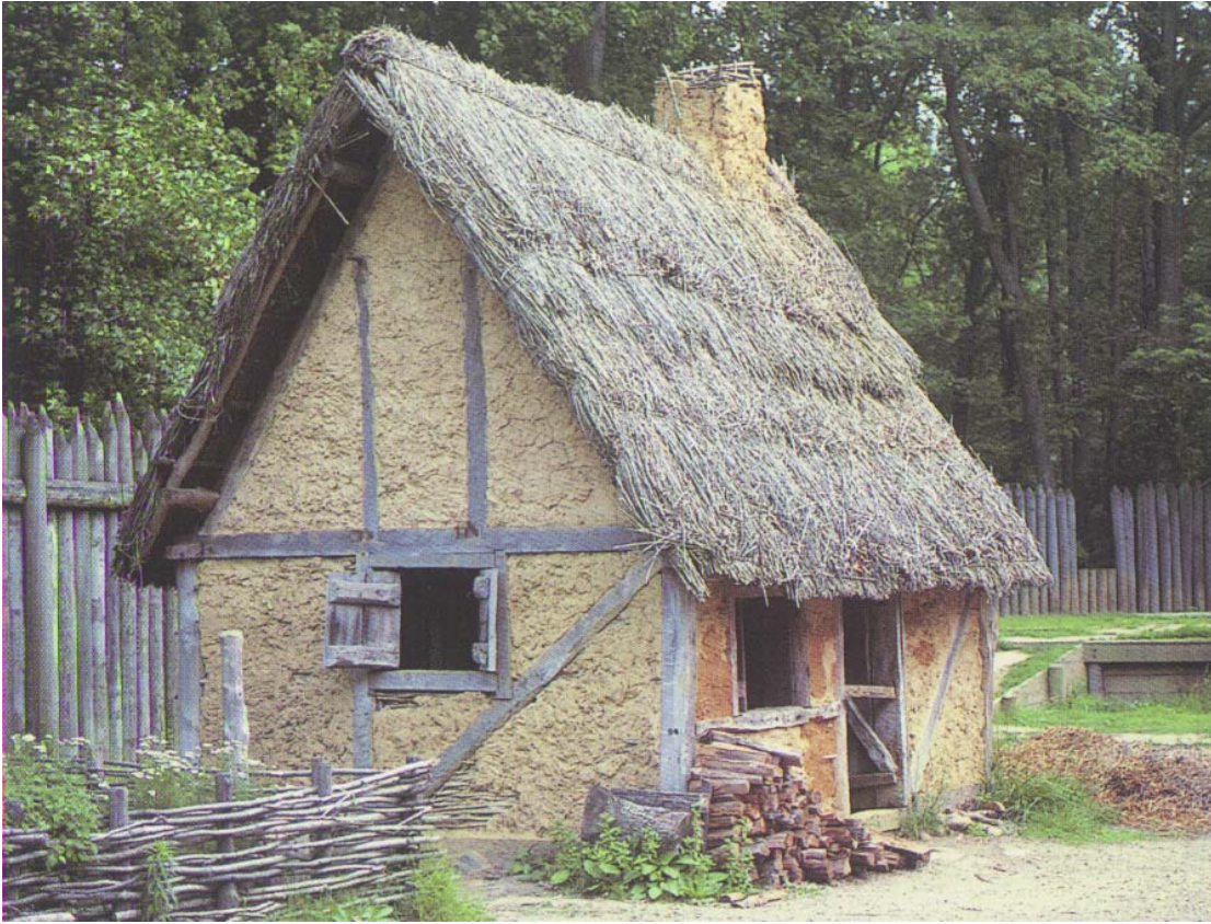
Figure 37: Dwelling unit at Jamestown
