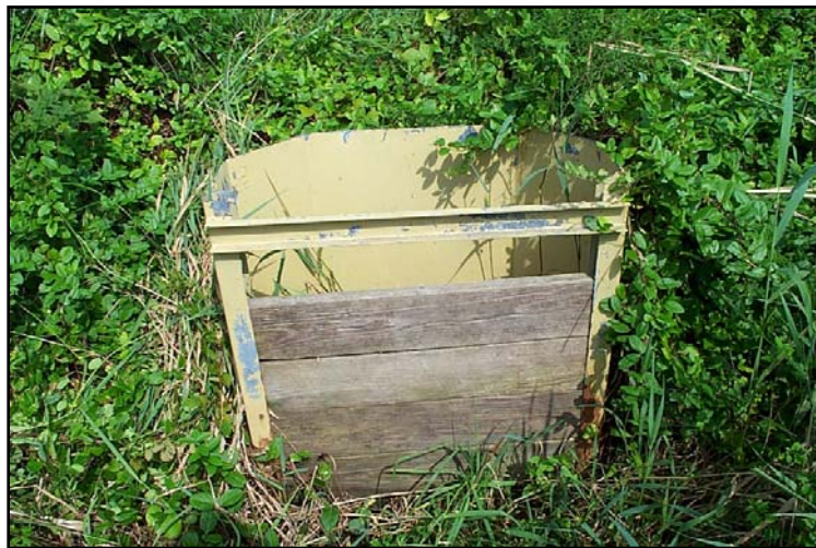
Figure 5. A flow control structure with removable wooded riser boards installed in a drainage ditch on the University of Maryland-Eastern Shore Campus.
