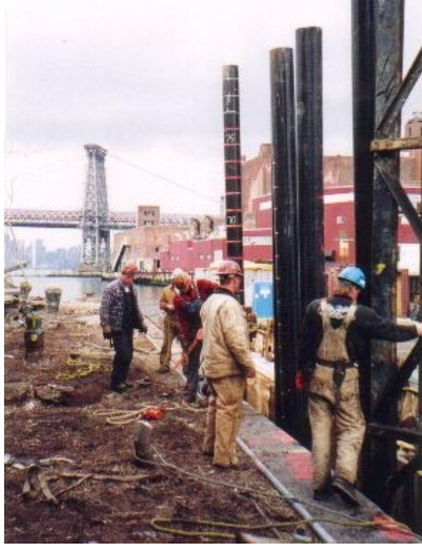
Figure 2-3: Lancaster Composites piling installation.
