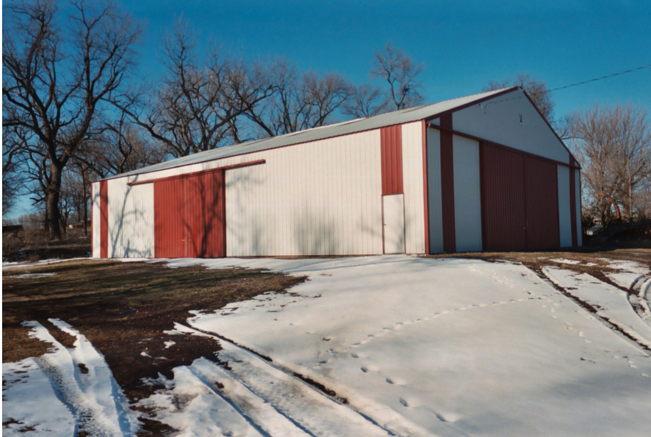
figure 45: quonset building : The largest building on site is the quonset building across Fountain Creek, on the north west corner, of the building complex. This metal building is the newest and largest building on farm. The building is built with a steel structure and faced with 3' metal sheets. This quonset contains most of the farm equipment used for modern farming.
