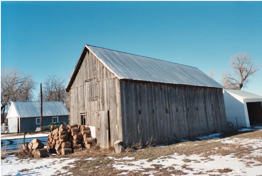
figure 42: original barn : Within the center of the old farm is one of the original barns of the farm, built in 1887. Now, the barn is used to store firewood. Old tree branches create the angled racks. The exterior is composed of a variety of different sized planks. Each side of the building has a series of small metal rectangles attached to the exterior of the building covering holes formed by time.
