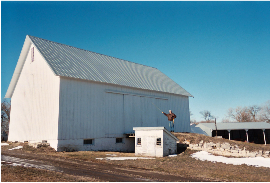
figure 41: big barn : The large white barn within the center of the outbuilding is the third major outbuilding on the site. The barn is constructed with moderately sized wood timbers and wooden pegs. This building also employs the use of ramps and the topography of the site. The building has two ramps on the west and east sides of the building, which allow for farm equipment to move through the building. The lower level of the barn is accessed from grade on the north side of the building. Currently the barn is not used for farming, but for storing an old boat.
