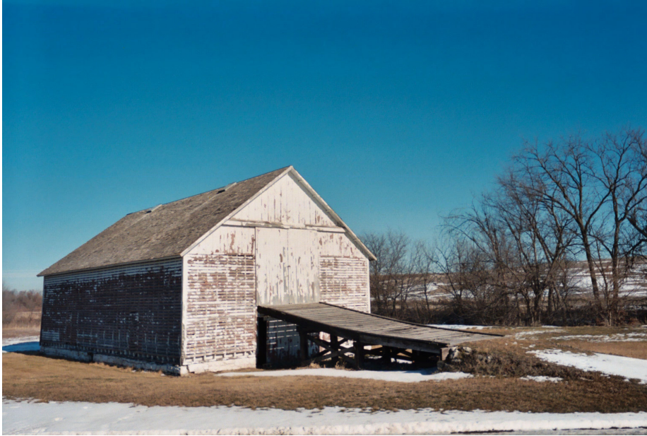
figure 39: ramped barn: This ramped barn is the first barn encountered upon entry to the farm. It serves as a figure piece for the outbuildings. The ramp is elegant as it moves from an earth bermed ramp and into a ramped bridged. The ramp currently is in need for repair and is unsafe to walk on or drive on. The exterior of the barn is constructed to let air freely move through, it is similar to a lattice. The barn is currently slated for demolition in the summer 2004.
