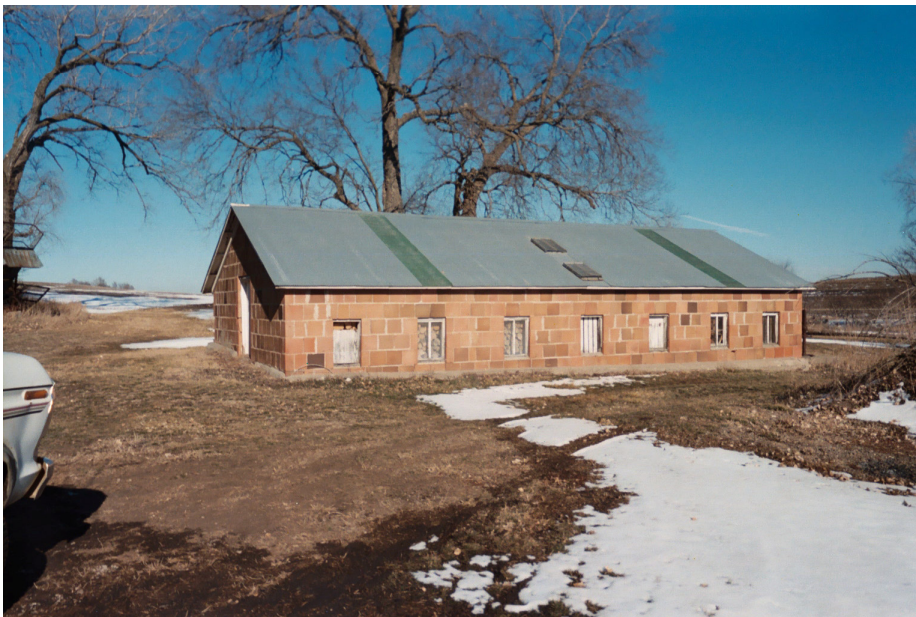
figure 46: hog pen : The old hog pen is the northern most building of the farm complex and is the farthest from the farmhouse. The building is low to the ground and is constructed of large bricks.
