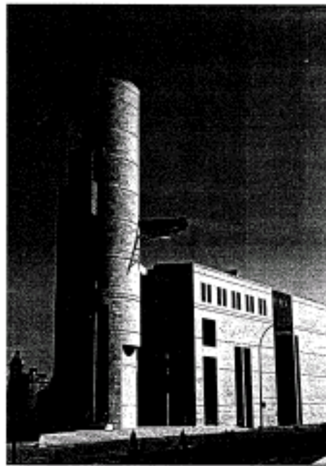
Main entrance facing Place Royale.
