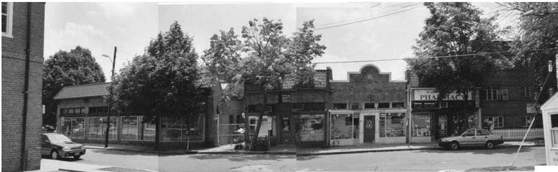
Figure 21 Panoramic of the north side of the site showing from left to right: the Chevy Chase Post Office, the Shoe and Luggage Repair Store, the Shoe Store, the Chevy Chase Pharmacy, and the Northampton Building. Source: Author's Files.
