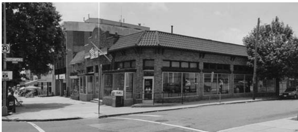
Figure 23 View of the post office and Moto Photo showing its Connecticut Ave. and Northampton St. facades. Source: Author's files.
