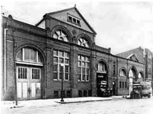
Figure 64 The original street car barn that eventually became the Charles Theater. Source: www.thecharles.com
