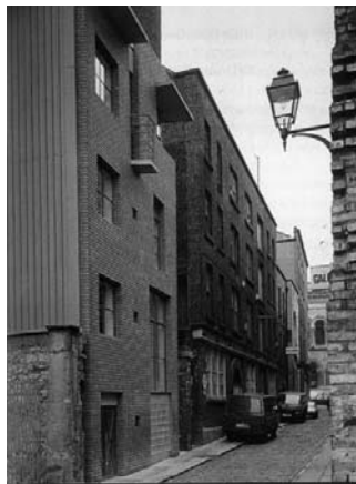
Figure 79 View of the façade of the archives, the only street frontage the IFC has. Source: Catherine Slessor.
