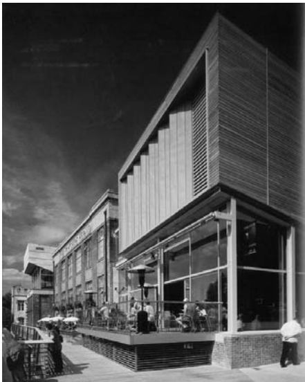
Figure 81 Cinema using wood and glass and containing a café/restaurant with outdoor seating. Source: Edwin Heathcote.
