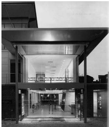
Figure 83 Entrance to the Tricycle Cinema in Manchester, England, showing the transparency of the façade, blurring the inside and outside. Source: Edwin Heathcote.
