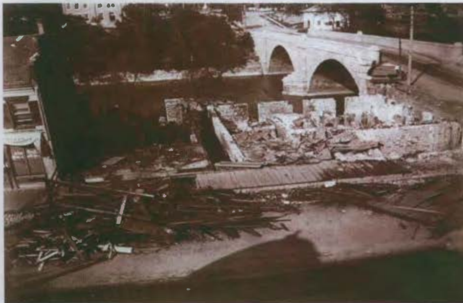
Before the new Elkader State Bank was built
