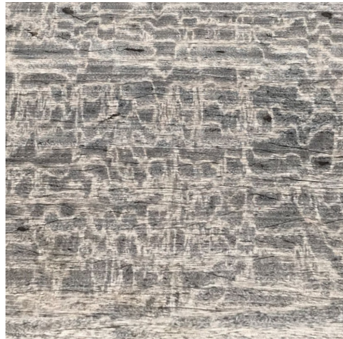
A wooden handrail’s grain pattern, visible after exposure to the elements.
