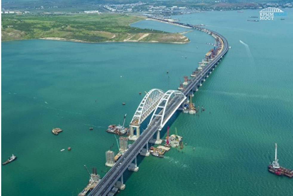
Fig. 2. Top view of the Crimean bridge
