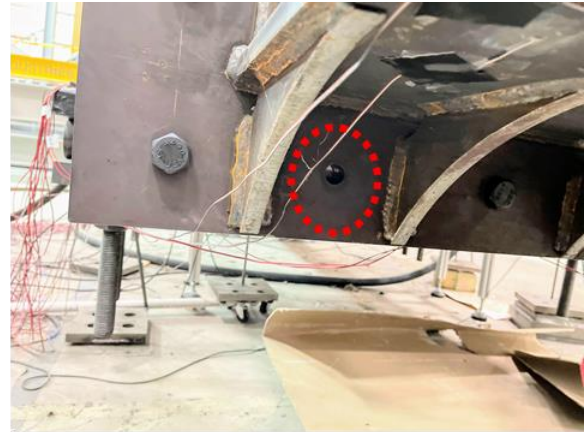
Figure 5-31. Example of the bolt failure locations.
