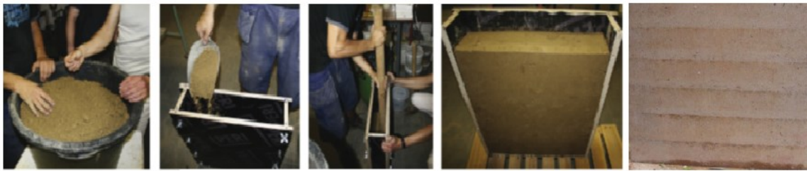
Fig. 1.1. The process of layer-by-layer RE construction [9].
