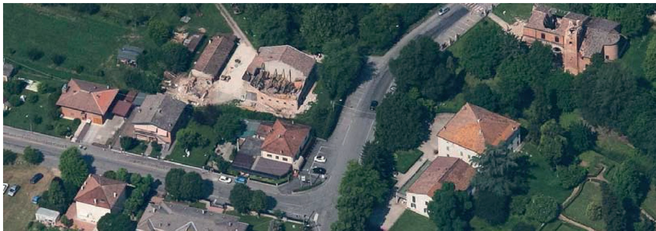
Figure 2 | Medolla, Modena. The roof, resting on long span walls, collapsed and directly contributed with its thrust to the out-of-plane overturning of the walls.
