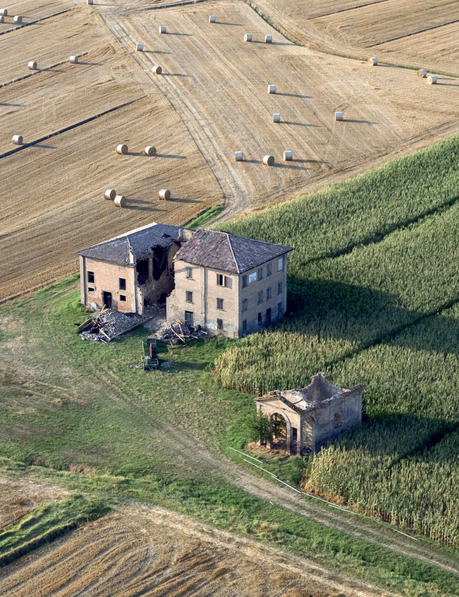
Finale Emilia, Modena. Tenuta Campa. The collapse of the timber roofs mainly caused the damages suffered by the rural dwelling and its annexed oratory.
