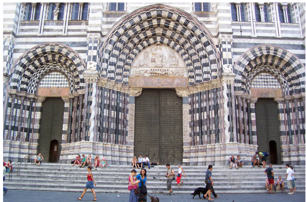
Figure 2. Façade of the cathedral in Genoa. It is composed of white marble, red limestone and green blocks of serpentinite. Picture courtesy of V. Sánchez Escribano.
