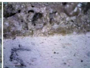
Pic. 20. Test 1b in cut
