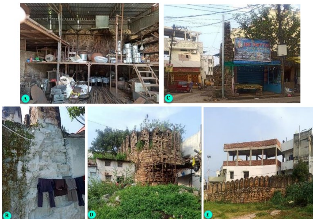
Figure 10. Isolated wall remains in different parts of Hyderabad. (A) Deteriorated portion inside a warehouse. (B) Fort found at the back of a residential quarter (C) Broken wall leading to a main road intersection (D) Intact bastion, part of wall. (E) Part of wall going through a cemetery
