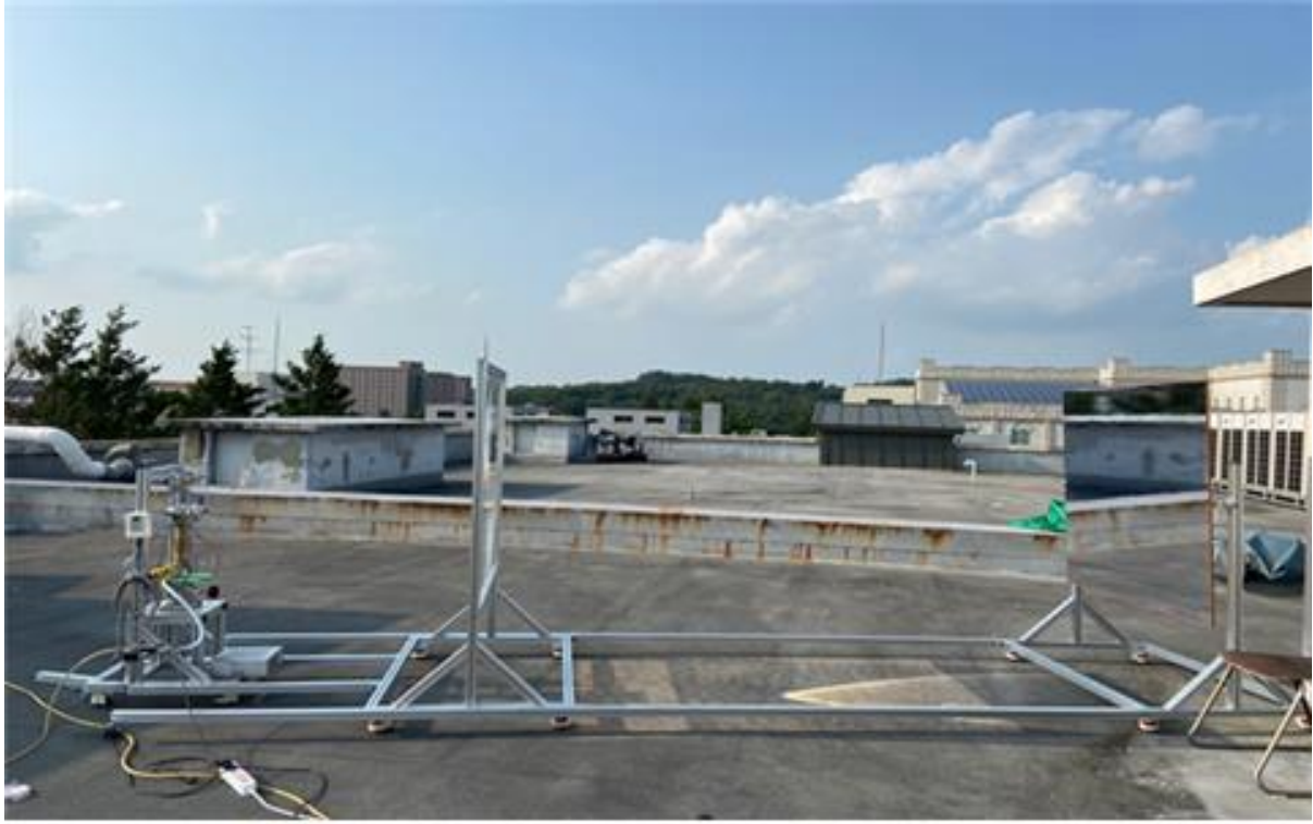
Fig. 3 Overall system configuration of the upscale equipment
