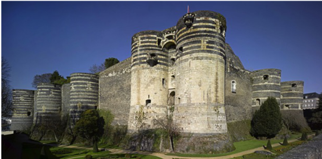
Figure 7.16: Banded Masonry at Angers Castle, Maine-et-Loire, walls from the 13th century. (Image: https://www.anjou-loire-valley.co.uk/diffusio/visit )
