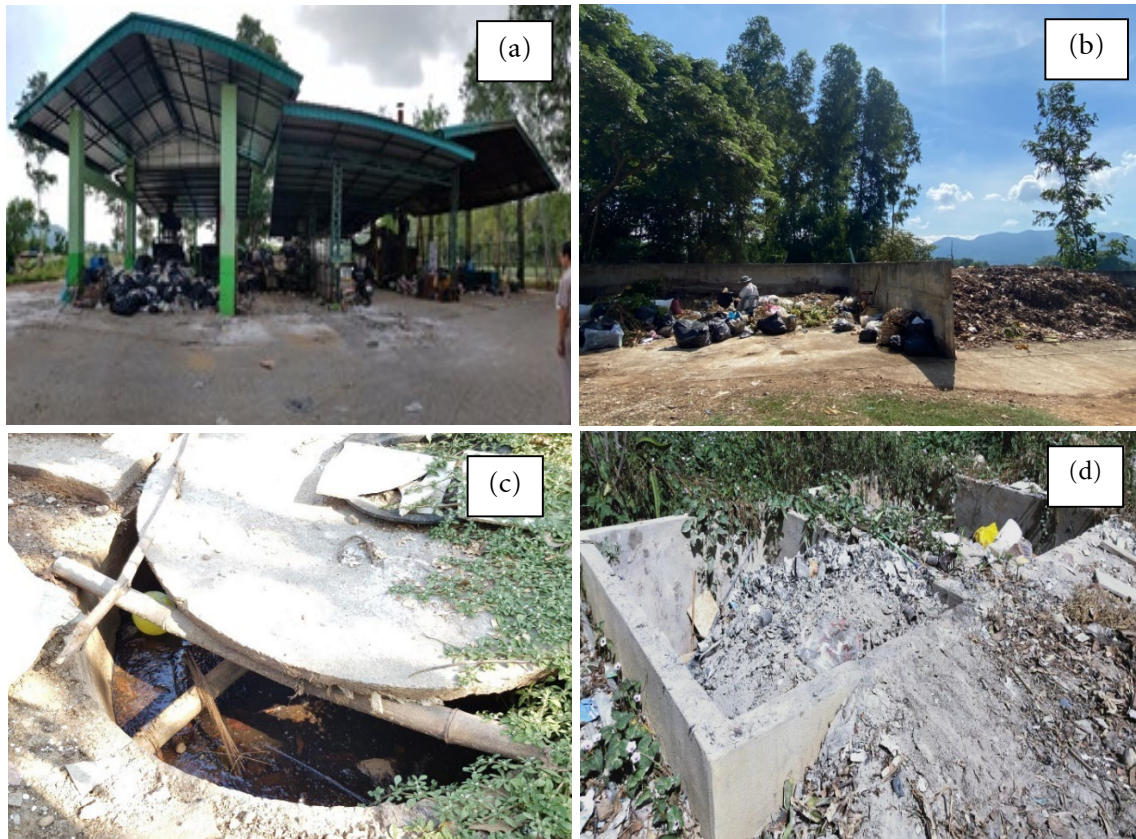
Figure 5 Pictures showing (a) waste disposal site, (b) composting area, (c) stagnant water from garbage and (d) ashes from the kiln.
