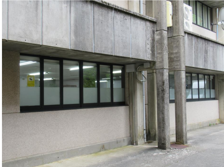
Figure 8. Building facade with windows.
