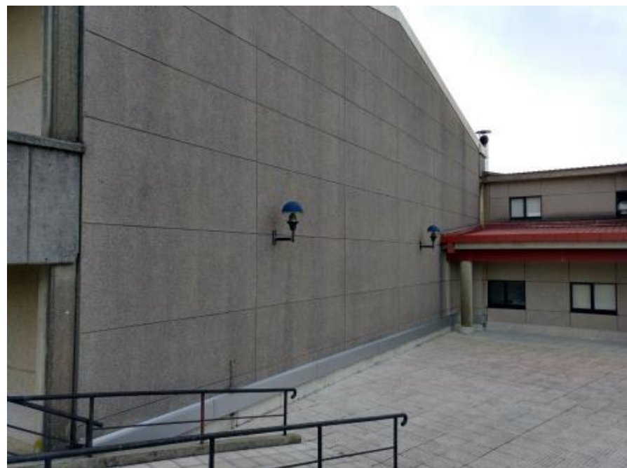
Figure 9. Building facade with no windows.
