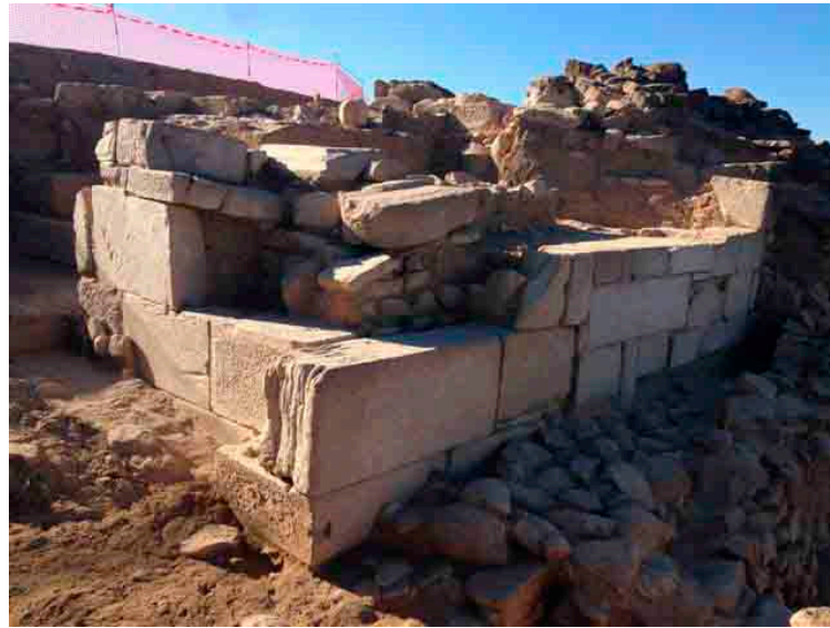
Figure 10. Photograph of the Roman-style wall, with five layers composed of large, irregular ashlars made from reused pieces.
