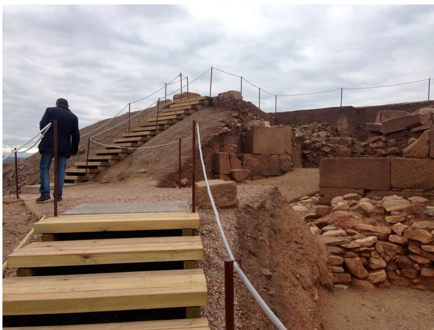
Figure 19. A wooden stairway which makes the visit user-friendly.
