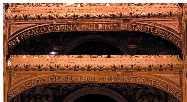
Figure 23. Before (A) and after (B) the intervention in the plasterwork of the tribune (cleaning and reintegration of volumes).
