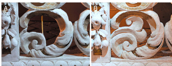
Figure 21. Volumetric reintegration (plaster + 25% lime paste) using a fiberglass structure. (A) Initial state and (B) reconstruction state.
