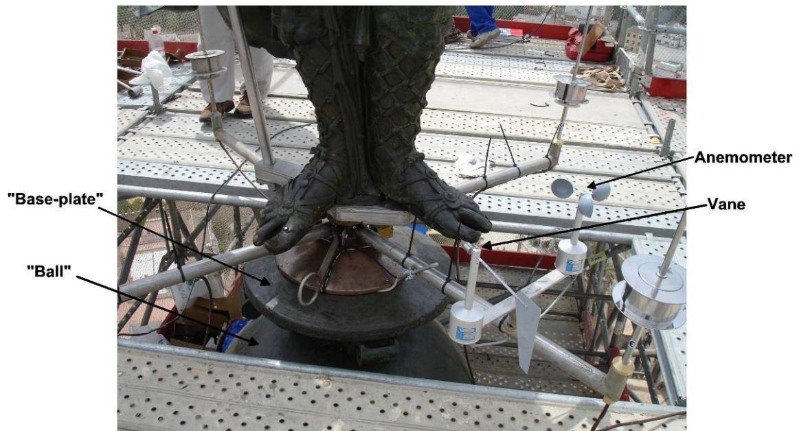
Figure 5. Sensors on the lightning rod support
