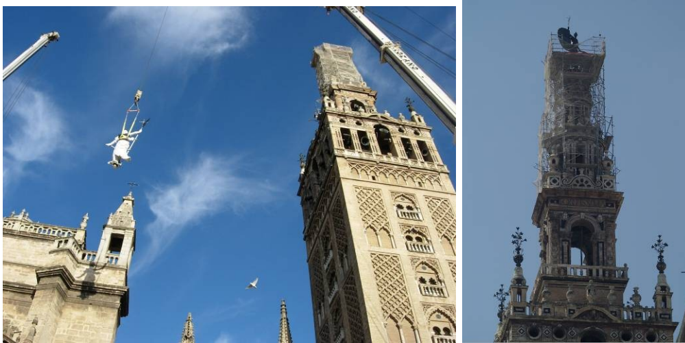
Figure 2. Mounting of the Giraldo atop the Giraldo Tower
