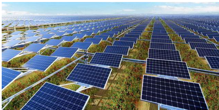
Figure 45. PV plant to feed the 150 MW electrolysis facility by Baofeng Energy [169]
