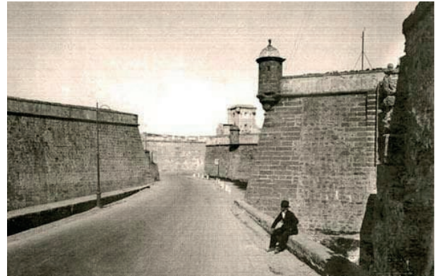
Fig. 7. Passage between counterguards and ravelins. (Source: Municipal Historical Archive of Cadiz).
