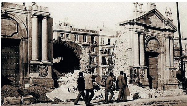
Fig. 6. Image of the since demolished Puertas del Mar when the sections of wall in which they were embedded had been taken down. (Source: Municipal Historical Archive of Cadiz).
