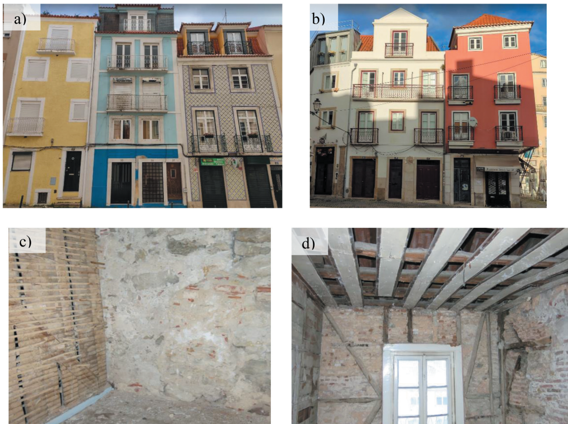
Figure 5. “Pre-Pombalino” typology: (a) and (b) example of building facades aesthetic; (c) “Tabique” in exterior walls supporting the timber floor; (d) “Tabique” in partition walls.
