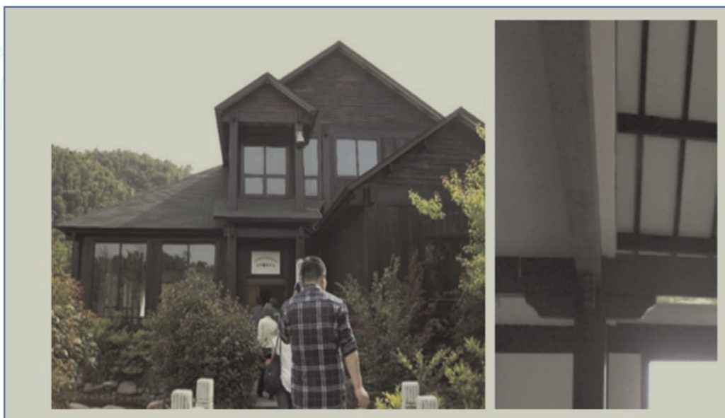
Figure 10. Bamboo house, Moso bamboo modern Technological Park, Anji, China (adapted from [35] with permission).
