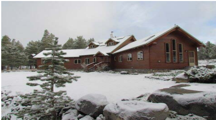
Fig.43 Photo of “Mountain Bluebird Lodge” California, house built in 2000-2001
