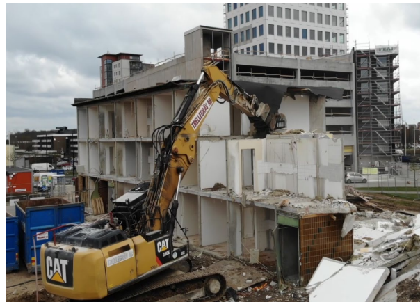
Figure 2. One of the Swedish donor buildings, during deconstruction.
