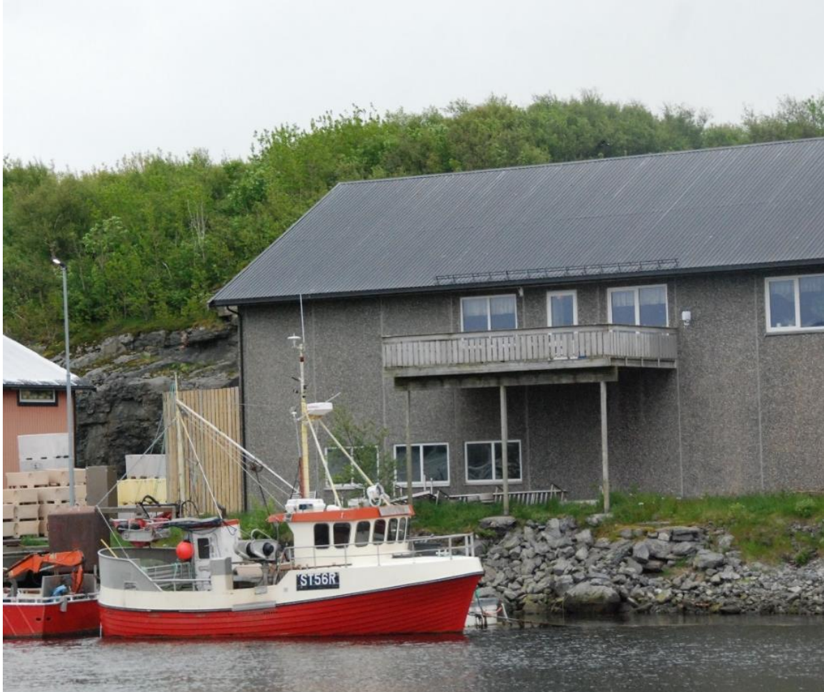
Figure 2. The balcony overlooking Roan fish handling facility, where the rails were mounted.
