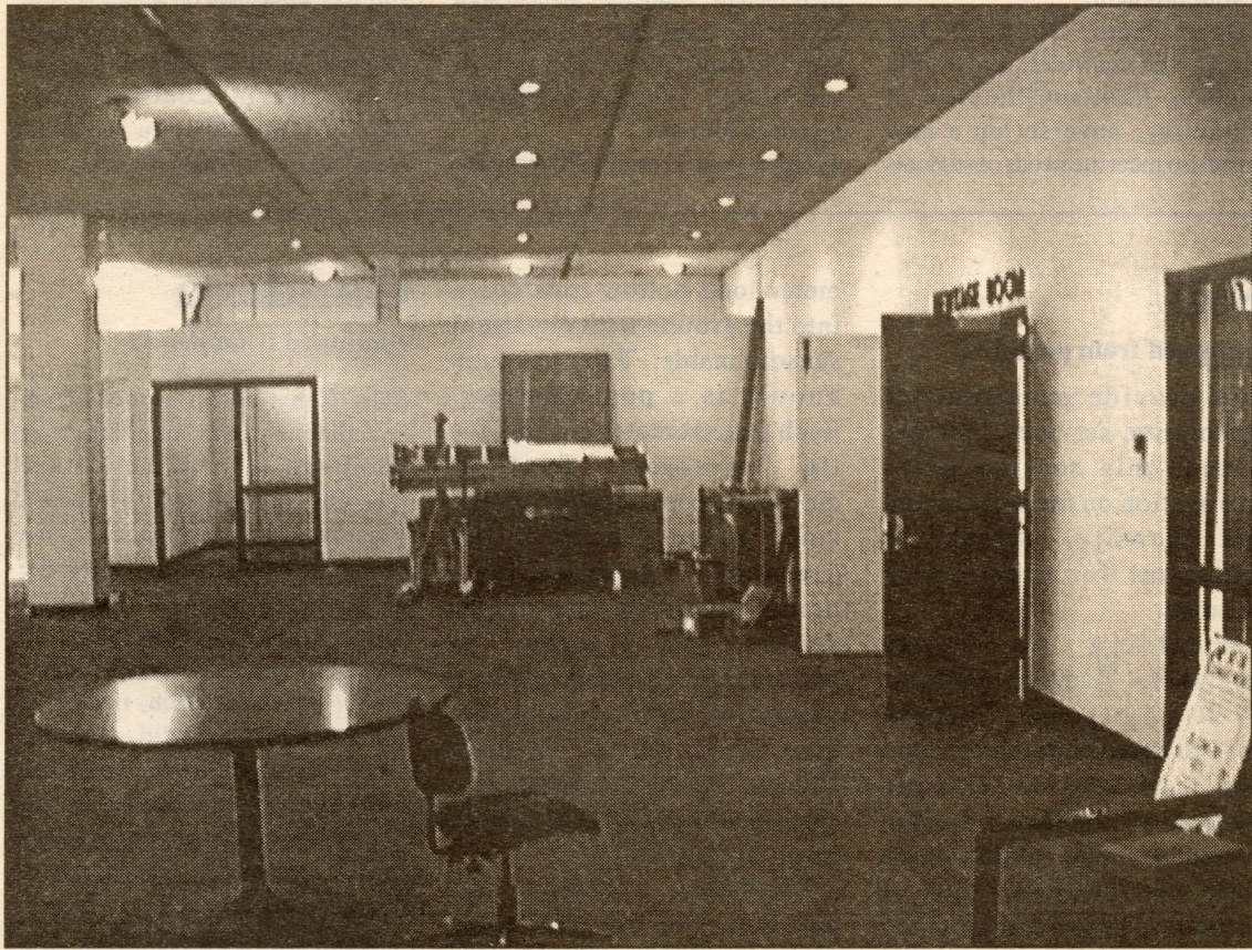
Cafeteria is emptied in preparation for remodeling.
