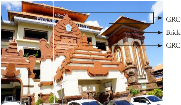
Figure 6. Facade of the Badung market. (Source: author, 2021)
