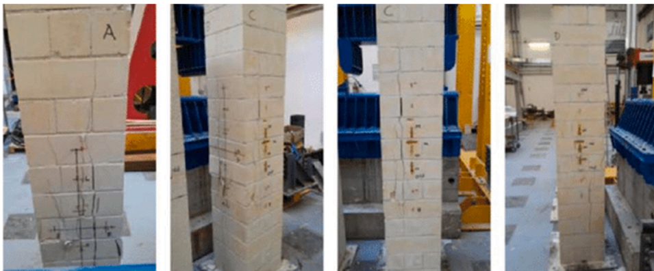
Fig. 1. Brittle Failure of Unconfined Column [26].
