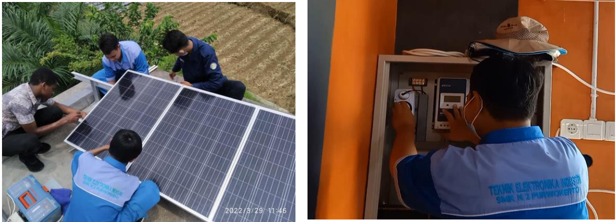
Gambar 4. Proses Pemasangan Panel Surya, Box Panel Inverter dan Controller
