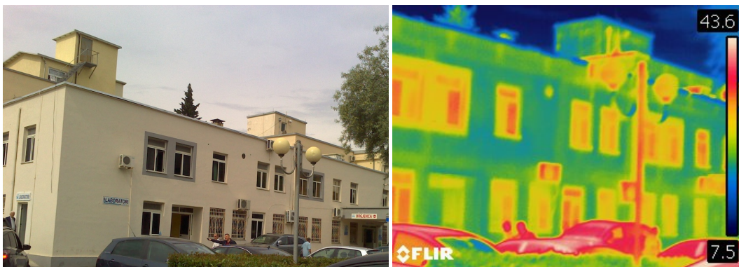
Figure 6. Image of façades from thermal camera
