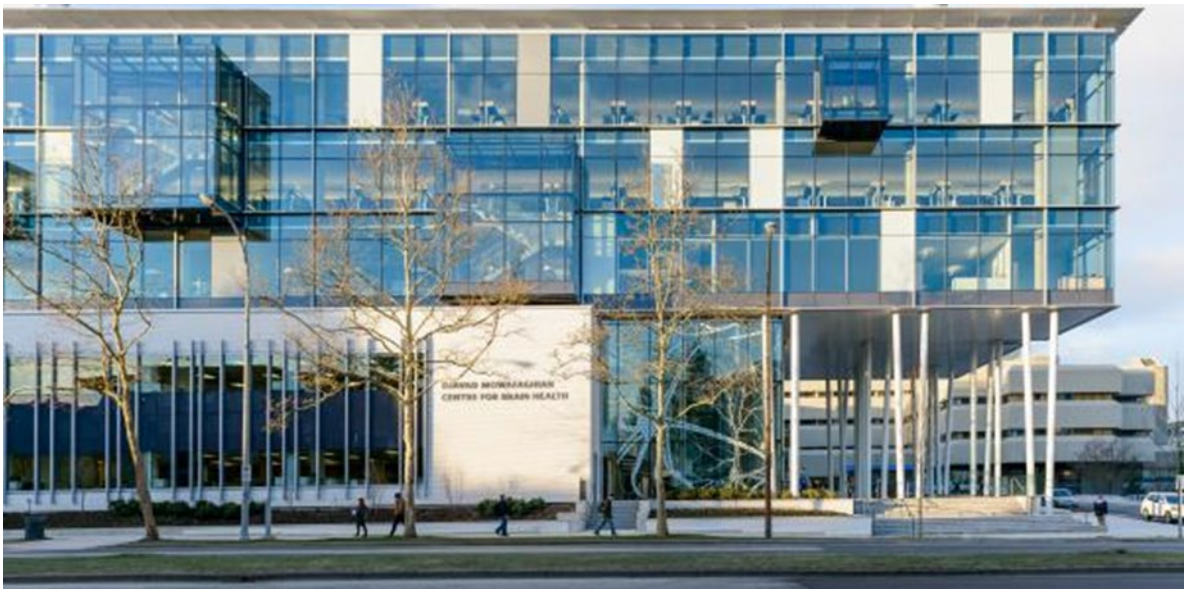
Figura 58. Vista exterior del Centre for Brain Health. FUENTE: www.stantec.com .
