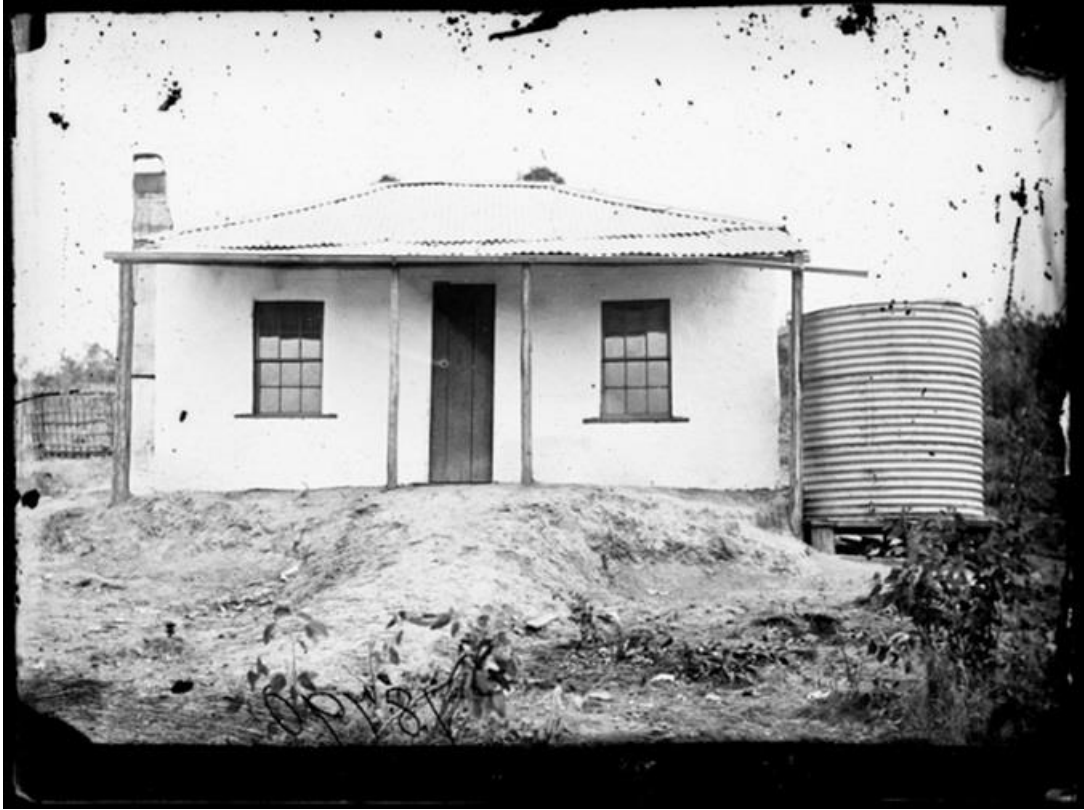
Figure 3.6: Whitewashed house with corrugated iron roof and water tank, Hill End (American and Australasian Photographic Company c.1871-1876). Source: State Library of NSW.
