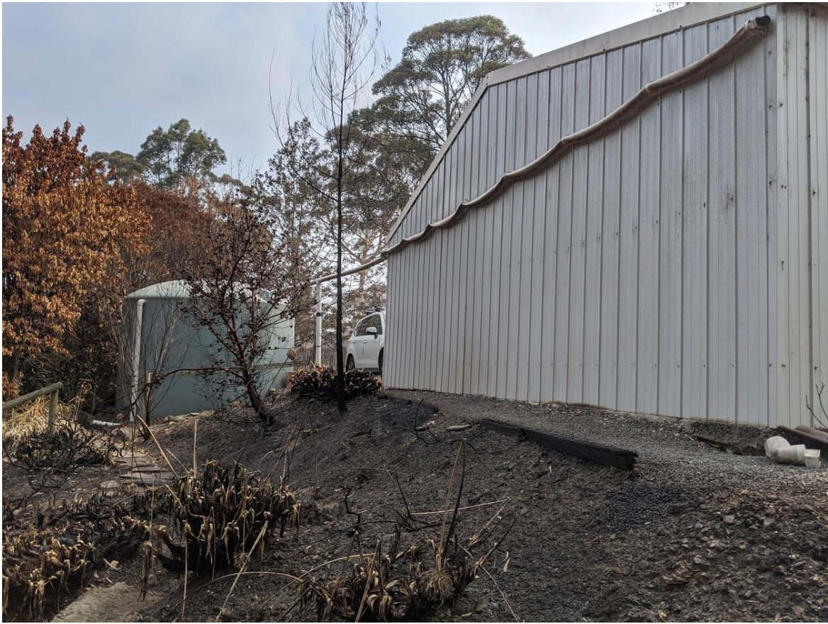
Effects of the New Year's Eve fire at home—surviving rainwater tank and melted water piping. Source: Author, 7 January 2020.
