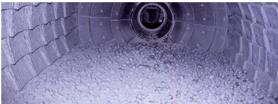
Figure IX.6 - The inside of a ball mill [Holcim Belgium (2013a)]
