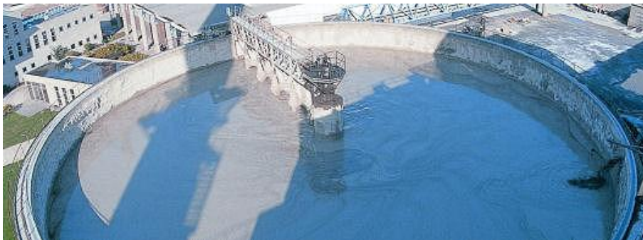
Figure IX.3 - The preparation of the slurry [Holcim Belgium (2013a)]
