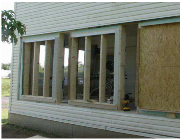
Three test bays in preparation.
