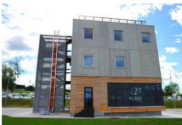
Eastern façade of KUBIK
