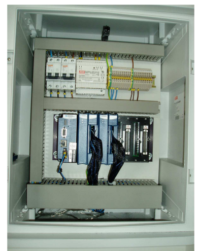
Box containing data acquisition modules
