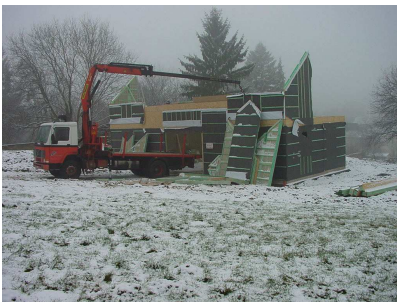
View of the facility during construction
