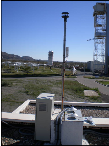
Meteorological devices and box containing data acquisition modules at the bottom of the mast
