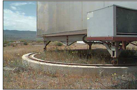
Detail of the rotating device
