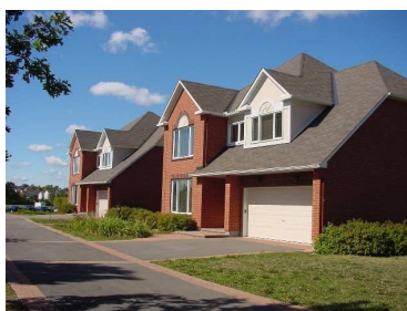
Twin Houses at the Canadian Centre for Housing Technology
