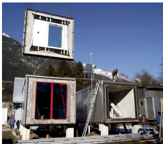
View of both test cells and replacement of one test facade
