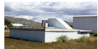
Exterior of the CETeB Test cell
