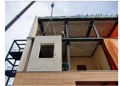
Prefabricated concrete façade element, developed with Norten-pH
