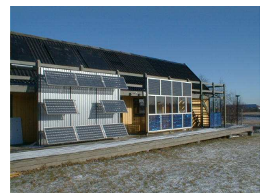
Test of pv systems.
