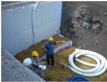
Earth to Air Heat Exchanger here in phase of construction (3 tubes, 10 m long each, 3 m deep). It was designed by eERG-PoliMI in order to maximize energy performances and to have a good layout for monitoring it.
