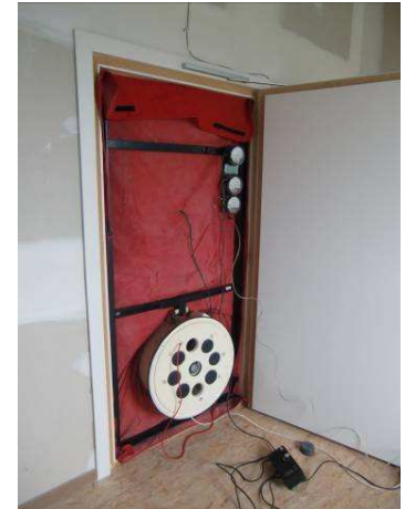
Air tightness test being performed in a measurement room in KUBIK
