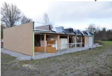
Facility during erection process
