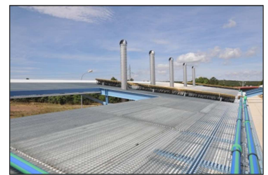
C-Ddl CEDER. Radiant night cooling system
