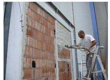
Insulating mortar projection.
