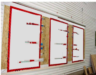
Test bays nearing completion.
