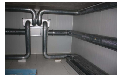
Interior of the CETeB Test cell
