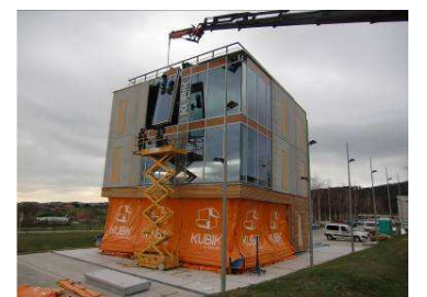
PV-Curtain wall developed by TECNALIA
