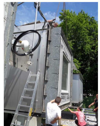
Mounting of test component (Project water:solution)
