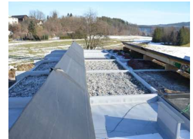
Investigation regarding roof shadings
