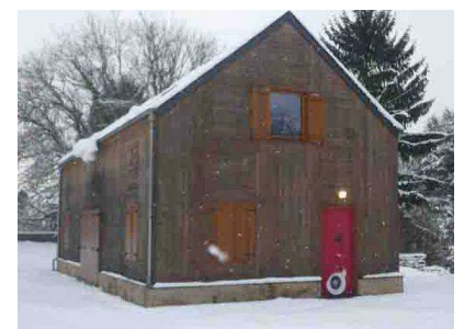
Blower-door test conducted on the building
