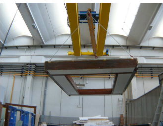
Installing the insulation frame for roof samples in ILARGI.
