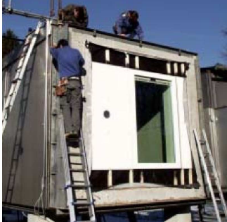
Mounting of test component (Project INTENSYS)
