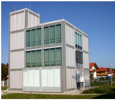
South-west view of the VERU test building.
