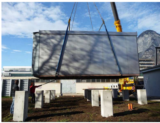
Placing the test cell at the UIBK test site
