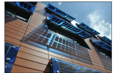
C-Ddl ED70 CIEMAT. PV shading devices
