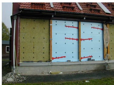
Measurement equipment at different heights and different interfaces in the building components.
