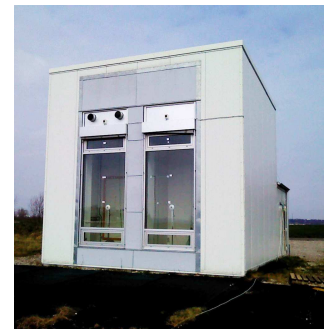
Present experimental set-up in the Cube. An intelligent façade (left), and unintelligent façade (right).
