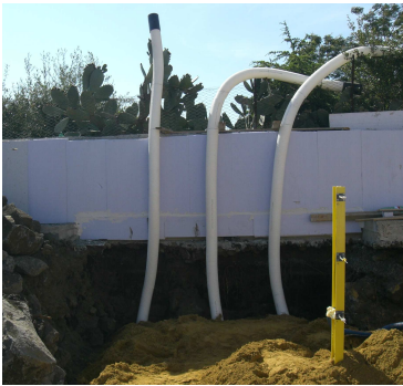
Earth to Air Heat Exchanger here in phase of construction (3 tubes, 10 m long each, 3 m deep). It was designed by eERG-PoliMI in order to maximize energy performances and to have a good layout for monitoring it.
