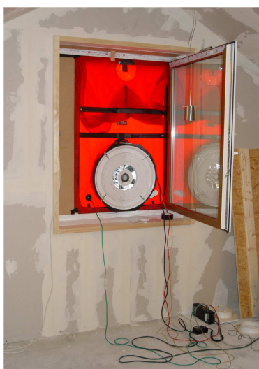
Blower Door device in attic
