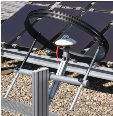
Radiation pyranometer with a circle to cast a shadow over the sensor in order to measure diffuse solar radiation.
