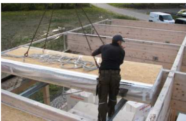
Mounting of roof assemblies
