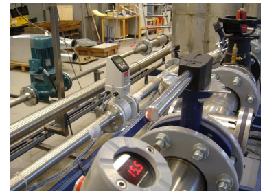
Test of circulation pumps.
