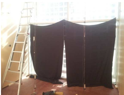
Figure 5. Mounting the inner solar protection
