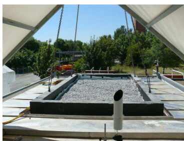
ILARGI: installing the roof covered by gravel to be tested inside the frame.
