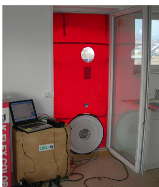
Airtightness test (blower door) in experimental houses.
