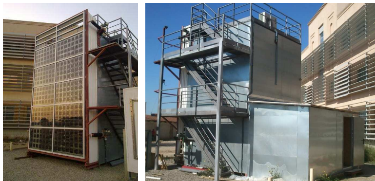
Figure 1. LOT test facility. Front and rear view.
