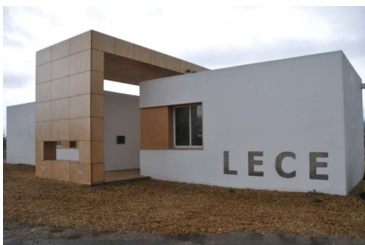
Monozone building. North face
