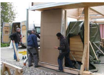
Mounting of wall assemblies
