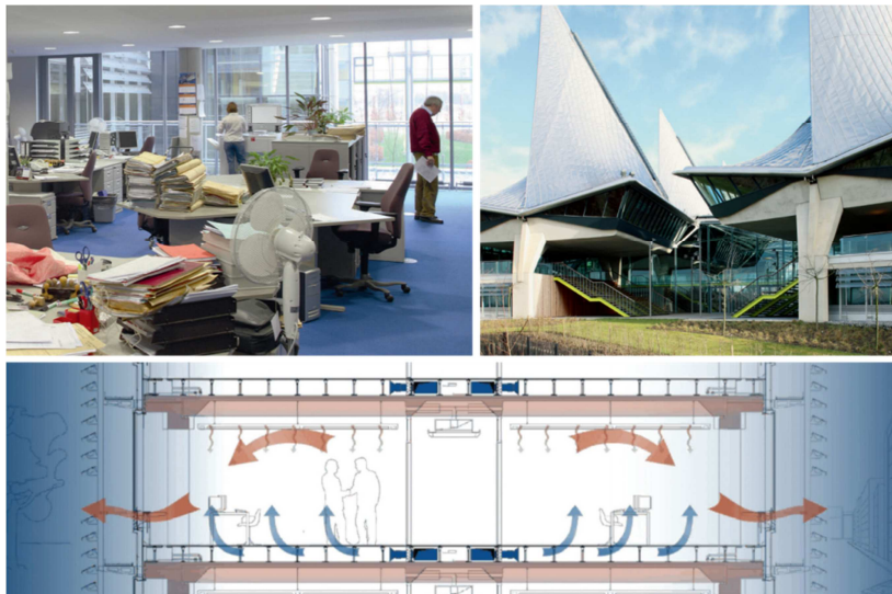
Figure 1.3: Courthouse Antwerp (Belgium) with mechanical night cooling (under floor ventilation and air supply via diffusers)
