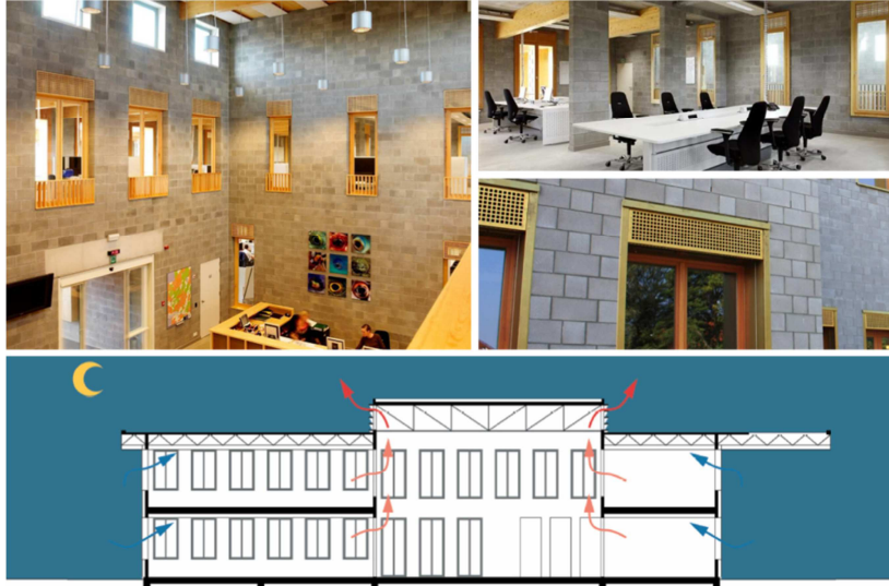
Figure 1.2: Police station Schoten (Belgium) with natural night cooling (stack ventilation and air supply via windows)
