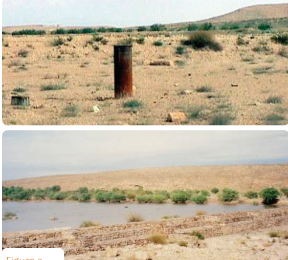
Figure 2. Gabion check dam (right) and recharge well (left). © M. Ouassar, M. Sghaier, M. De Boever, D. Gabriels
