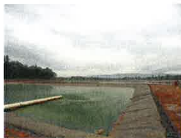
Figure 3. Picture of the wastewater stabilization pond (WSP) that treats the wastewater from Jimma University Technology campus.
