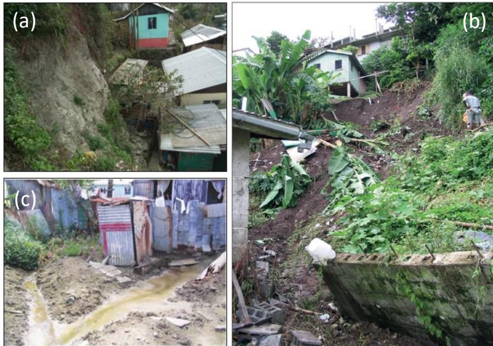
Figure 1.2: Examples of informal housing affecting land stability. Panels (a) and (b) show examples of unsupported cut slopes, respectively, in DumsiPakha (Kalimpong, India) and Saint Lucia (Caribbean). Panel (c) shows the effect of the lack of water management in an informal community of Saint Lucia (Caribbean). Source: the AGU Landslide Blog ( https://blogs.agu.org/landslideblog/2016/03/14/managing-urban-landslides-1/ , last access: 21 November 2020) and the community-based project Mosaic (Management of Slope Stability In Communities; Anderson and Holcombe, 2013).
