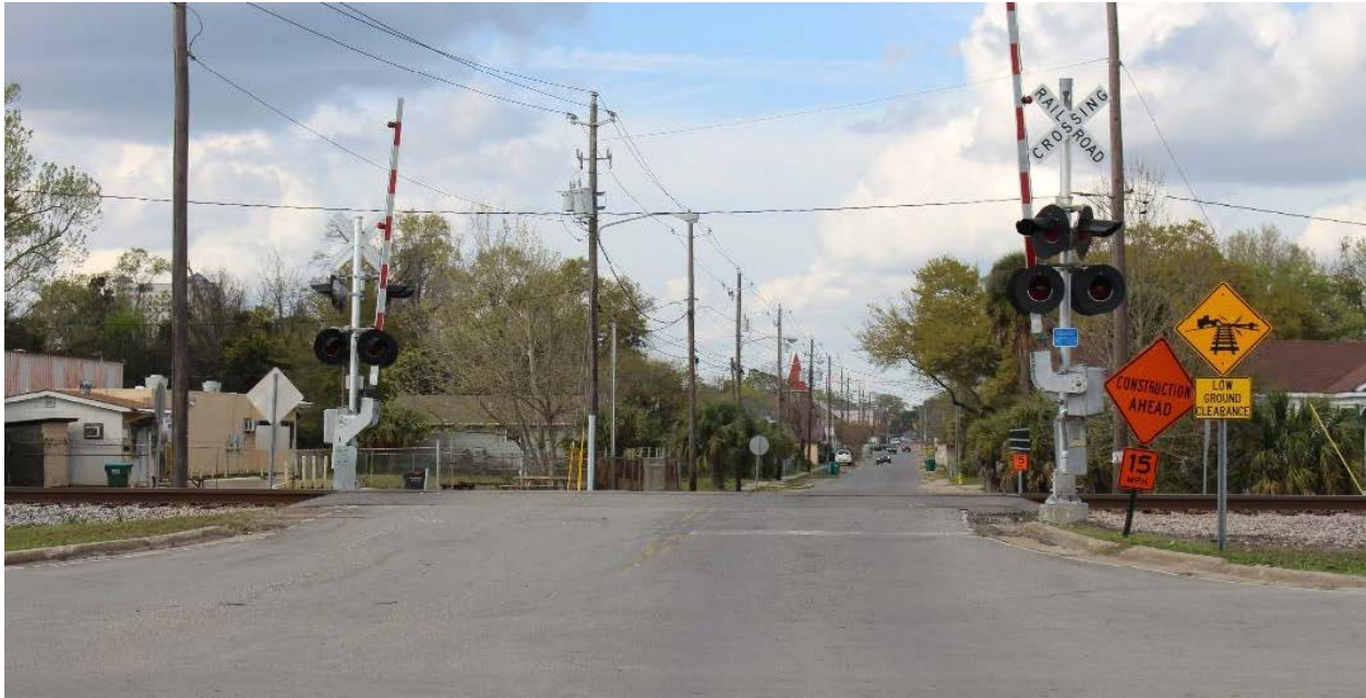
Figure 29. Main Street Crossing and Low Ground Clearance Sign in Biloxi, Mississippi [37]
