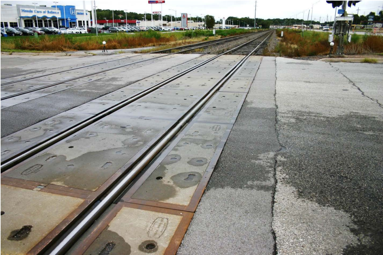
Figure 92. East Approach of Crossing 817404F
