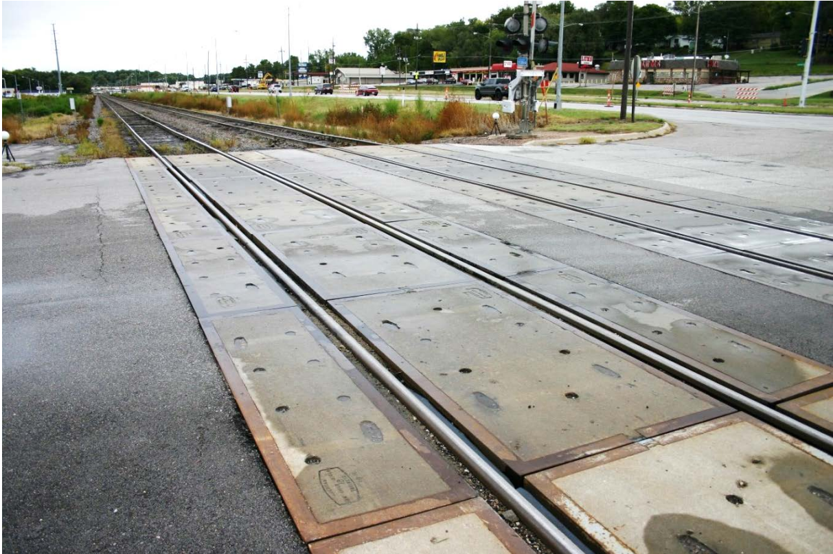
Figure 91. West Approach of Crossing 817404F
