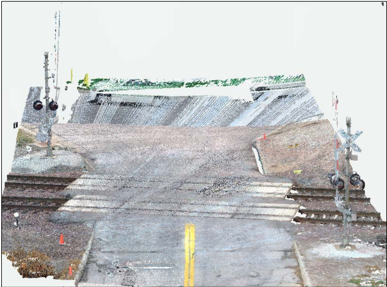
Figure 108. Crossing 817405M FARO Scan Front View
