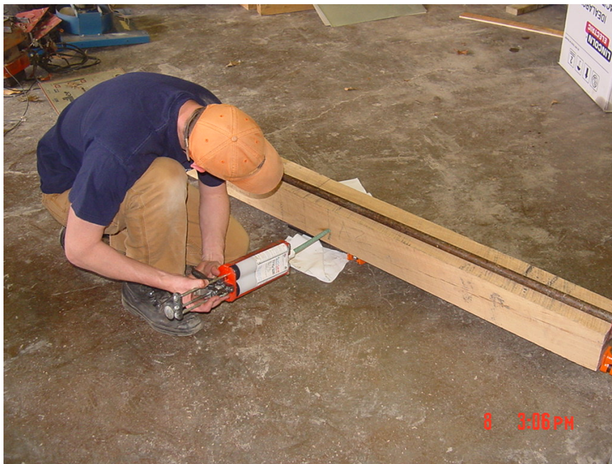
Figure 27. Photo. Injection of adhesive.
