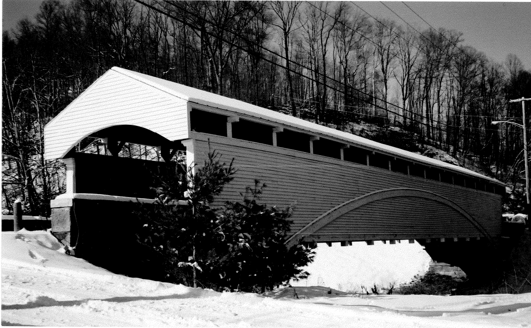
Figure 1. Photo. Barrackville Covered Bridge, Barrackville, WV.
