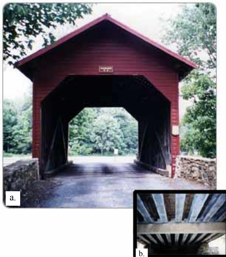
Figure 3. Photos. Roddy Road Covered Bridge (a) rehabilitated with steel I-beams (b), Frederick County, MD.
