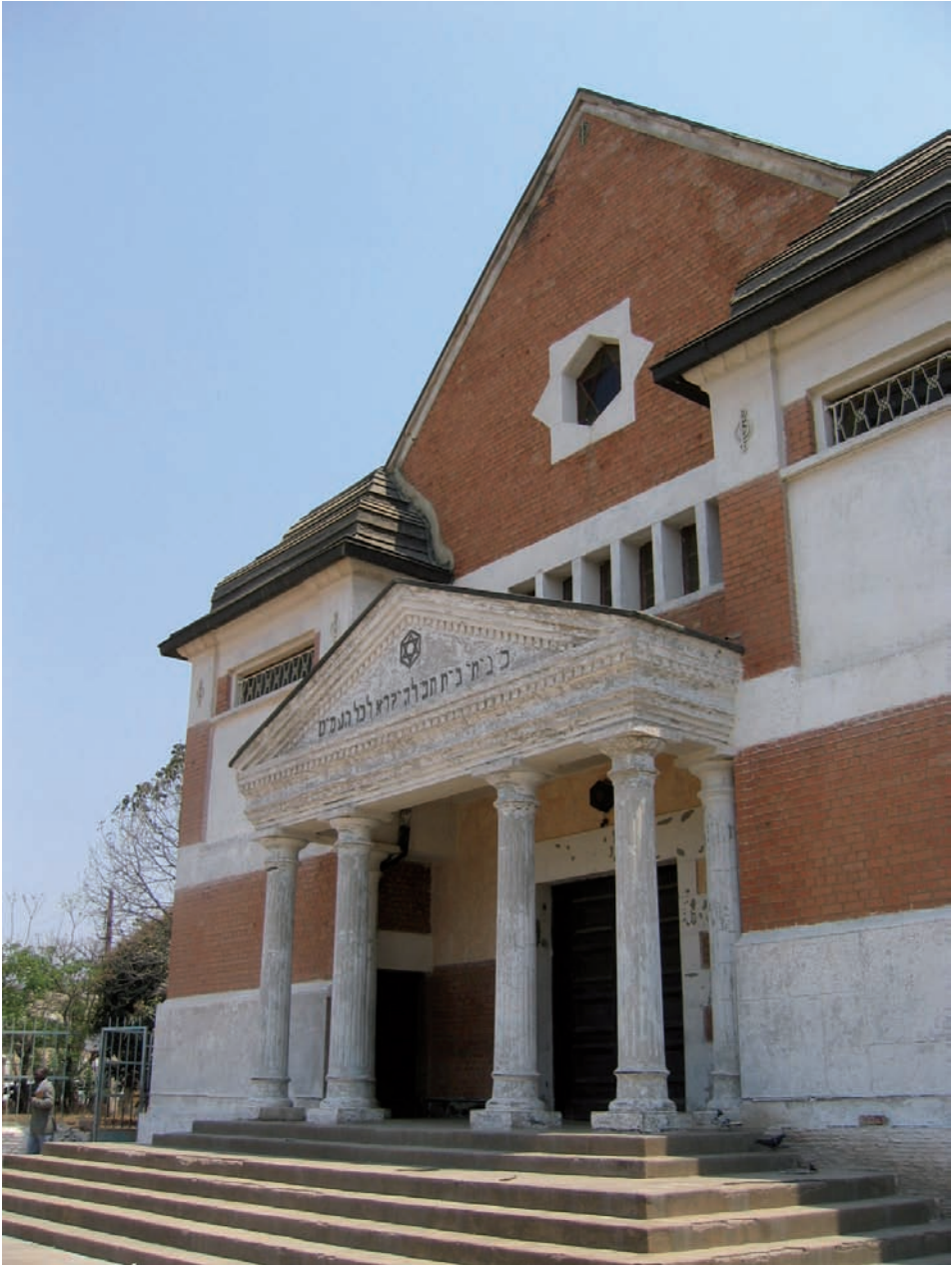
Fig. 6: Synagogue, Lubumbashi, arch. Raymond Cloquet, 1929 (photograph Johan Lagae, 2005)
