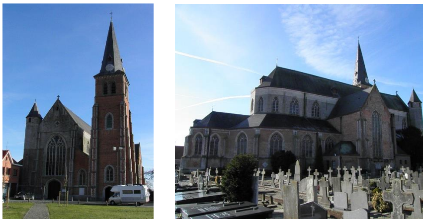
Figure 6.1: Church of Our Lady in Watervliet, Belgium.
